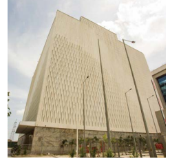
NTT Data Center – Chennai, India.
