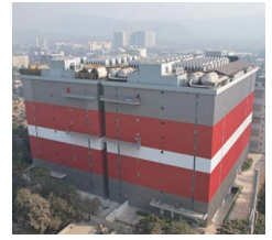
NTT Data Center – Mumbai, India.
