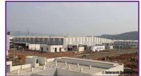
Khalapur plant(K2&K2) IGBC Green Factory Building Provisionally Certified- Platinum Rating
