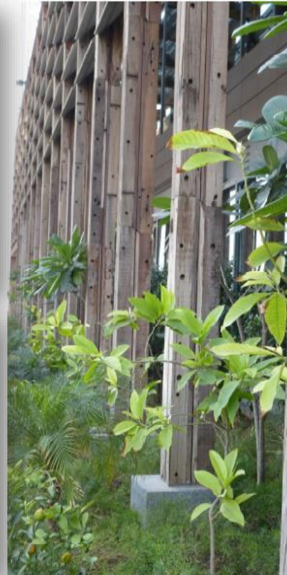
Use of railway sleepers bought from railway auction
