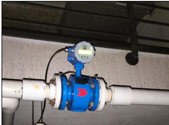
Water meters for Domestic water (treated lake water), HVAC & treated water for irrigation
