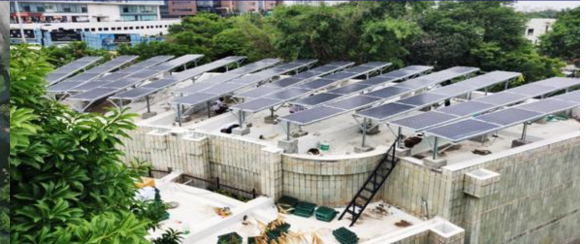
INDIA'S FIRST 140 kWp BIFACIAL SOLAR PV
