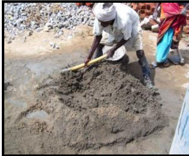
Hand Mix Concrete
